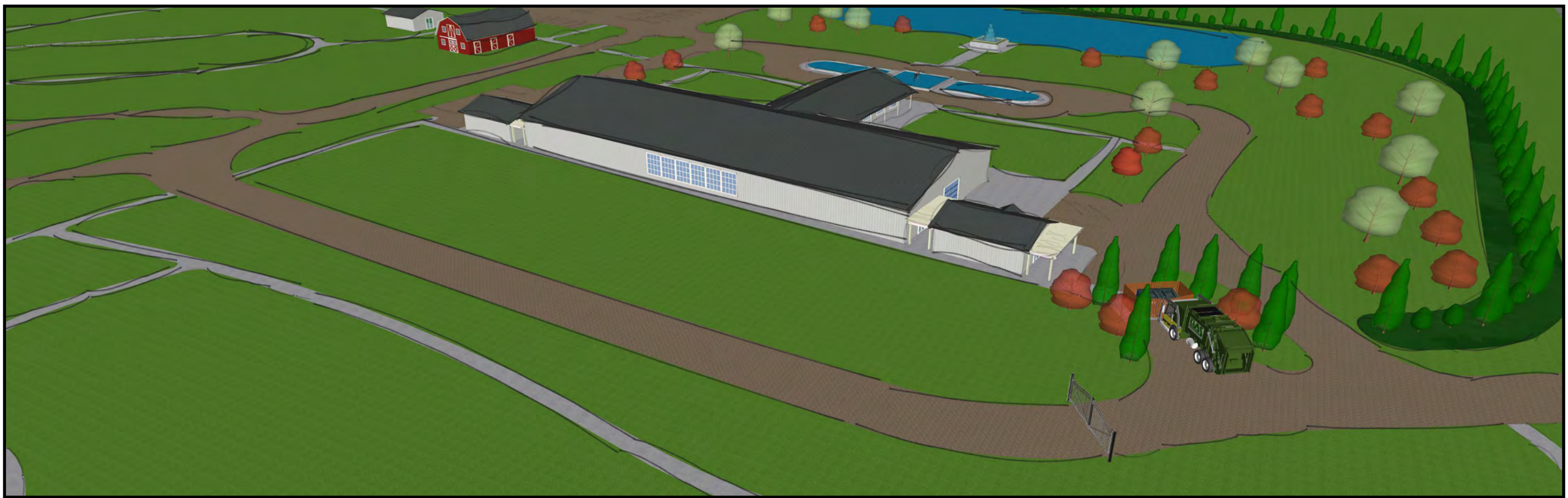
View of Rear of Main Facility
